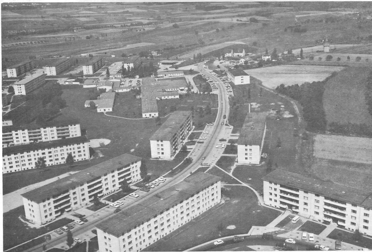
View of part of the Bitburg AB housing area and base hospital
