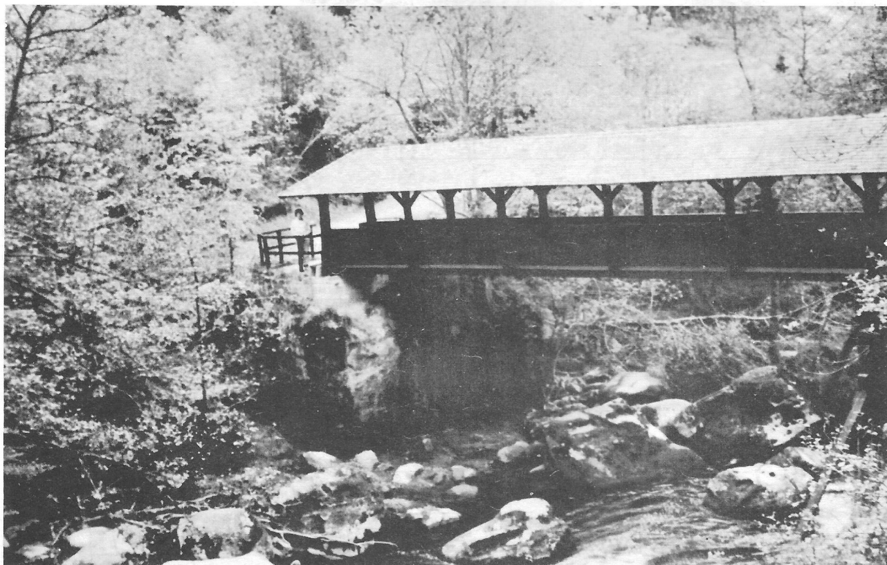
This covered footbridge crosses the Pruem River at Irrel about five miles from Bitburg. It is the starting point for a network of hiking trails.
